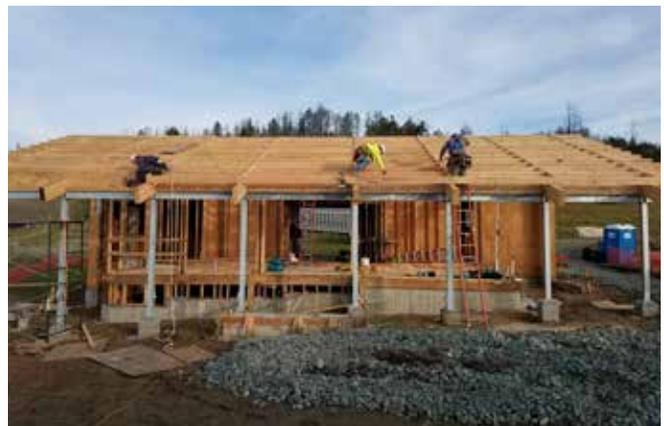
In rebuilding structures burned by the 2017 Tubbs fire, the design team proposed simple building typologies to minimize the sites where embers could collect—a deterrent against future structure damage.
